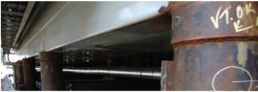
■ Figure 3. Inspecting piles attached to skid with slip rings for Saturn 1, 6500 hp (4849 kW) KBZ/6 compressor package.
