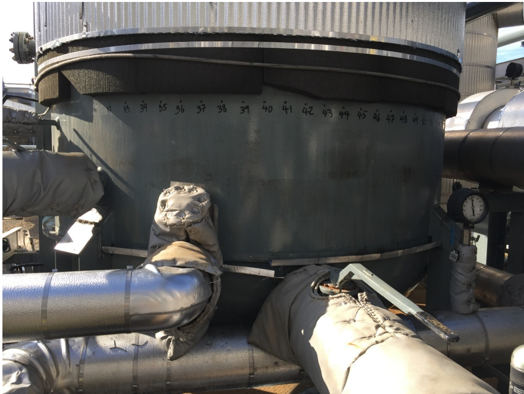
Figure 3. Location of vibration measurements on the shell of the oil separator
