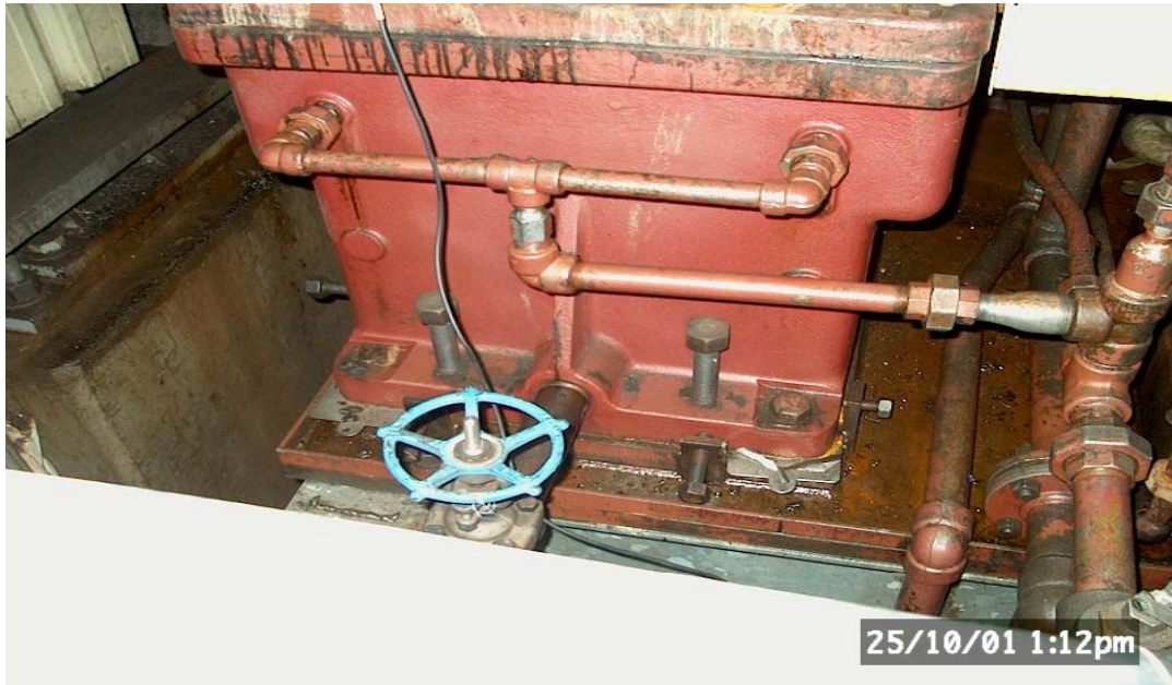
Picture 4: Gearbox base on the south side.
