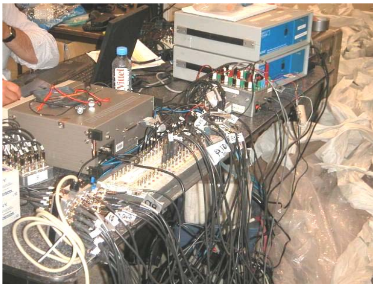
Figure 3. Dryer and calender stack monitoring equipment 32 vibration and 2 tachometer channels.
