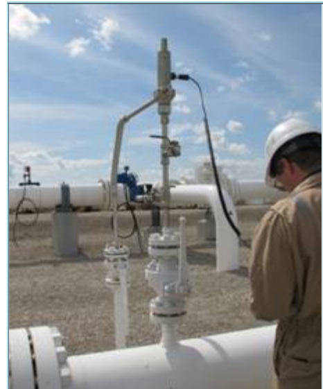
Vibration Audit on Small Bore Piping
